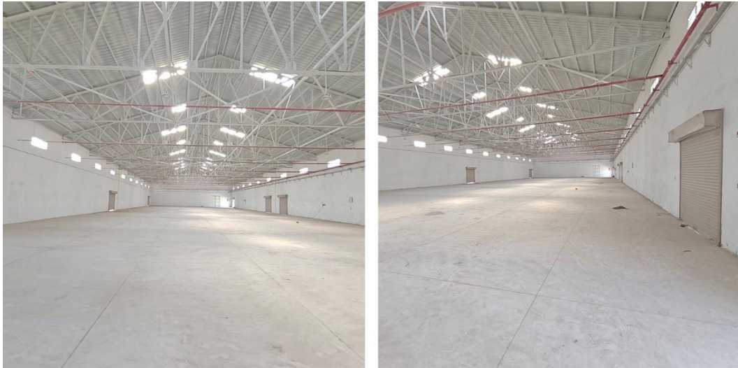
Inside View of Warehouse
